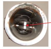
The clip must be removed with special tools to remove the heater through the tubing.
